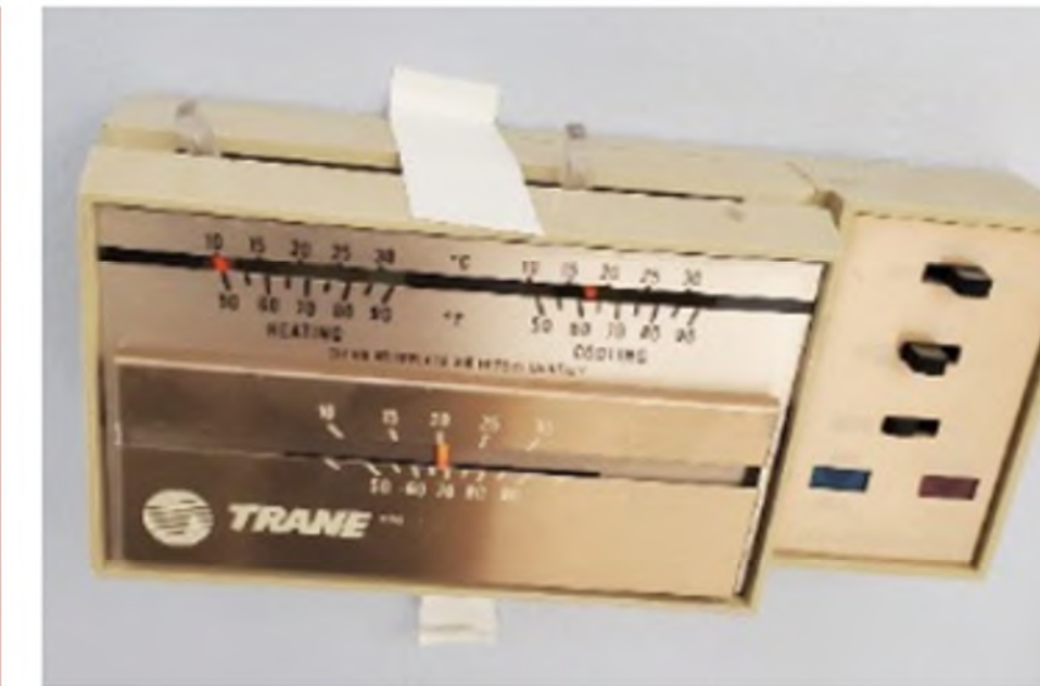
Typical HVAC Controls at MiSci
