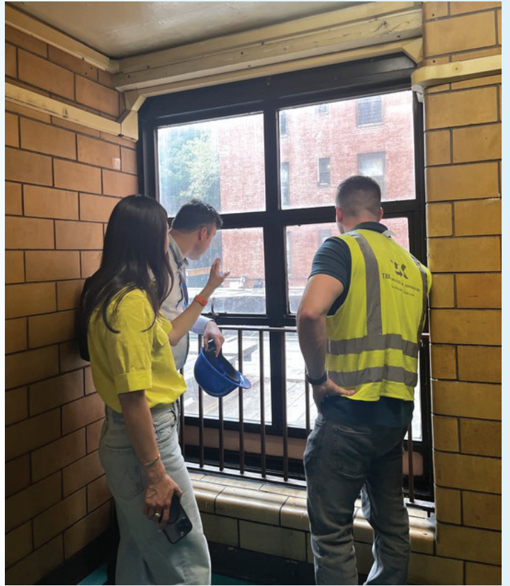
A walkthrough we held with tenants, NYCHA, and NYPD at Vladeck Houses to address scaffolding and security issues.
