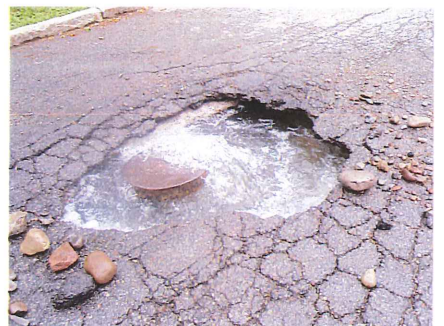
Comstock Ave. water main break 2014
